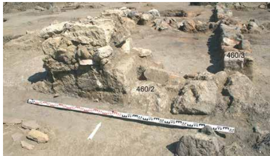
Fig. 9. Western part of the south wall (460/2): foundation and socle of the masonry. View from the SE.
