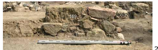
Fig. 42. Feature 169, faces of the middle part of the foundation: 1—north face (and SE corner of room 4 of building 460); 2—south face.
